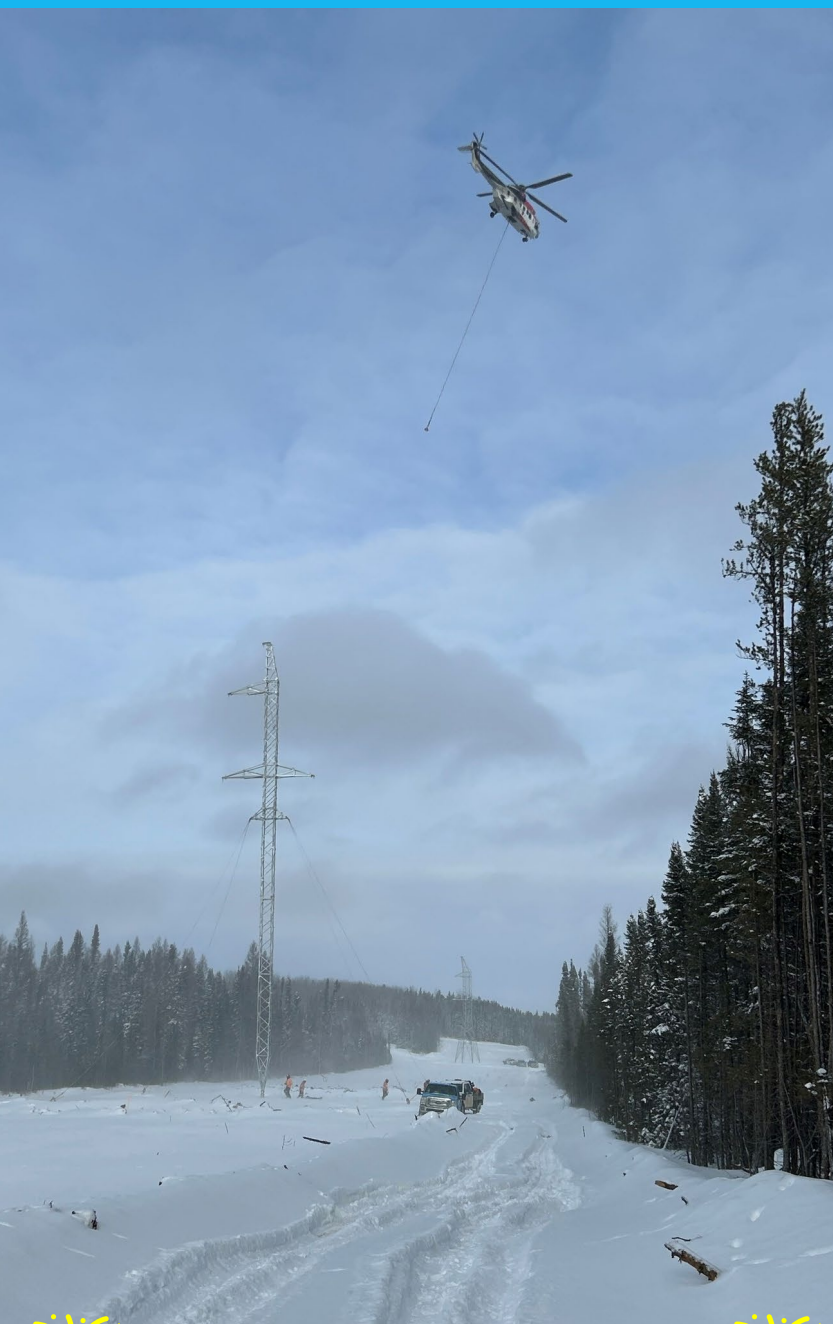
A four-legged tower (otherwise known as a self-supporting tower) in November on the Wataynikaneyap Power Project.
