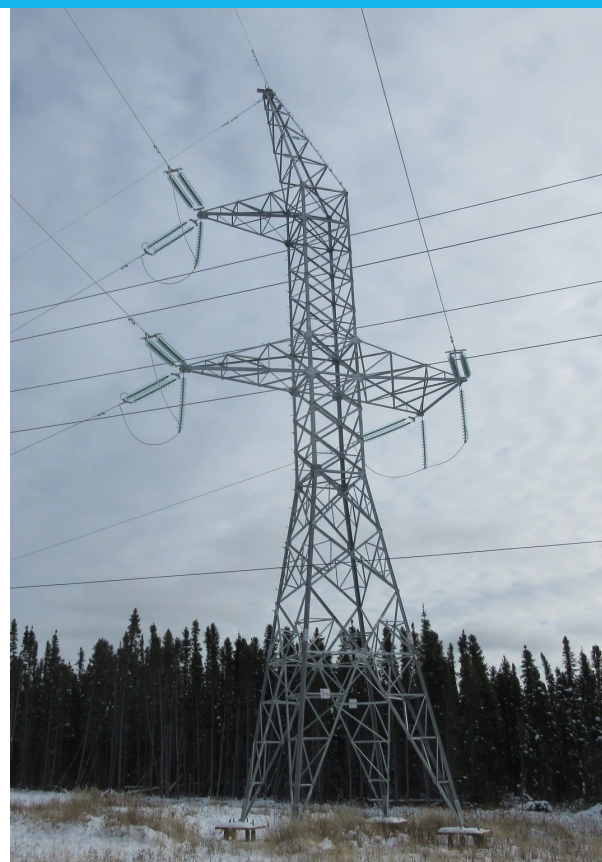
A four-legged tower (otherwise known as a self-supporting tower) in November on the Wataynikaneyap Power Project.
