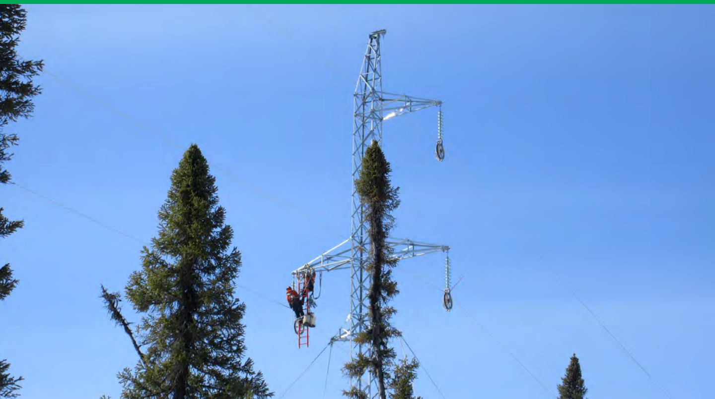
A powerline technician on a ladder attached to the tower arm, is preparing to hang a pilot rope for pulling conductor (wire) between Kingfisher Lake and Wawakapewin First Nations in March.
