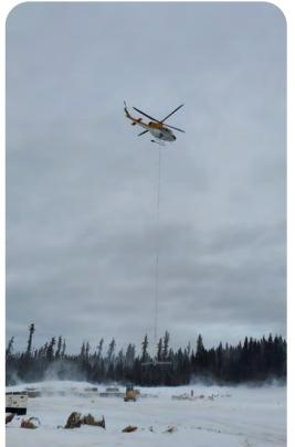
A Wiskair helicopter moving tower parts for the Wataynikaneyap Transmission Line at the Pipestone Camp.
