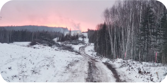
Obish Construction – Segment PQ Line Clearing
