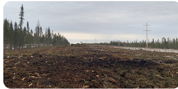
Missabay – Right of Way Clearing on segment BC.
