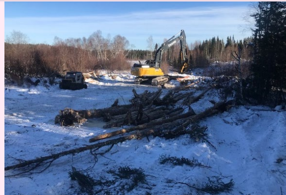
An excavator installing corduroy on a soft spot.
