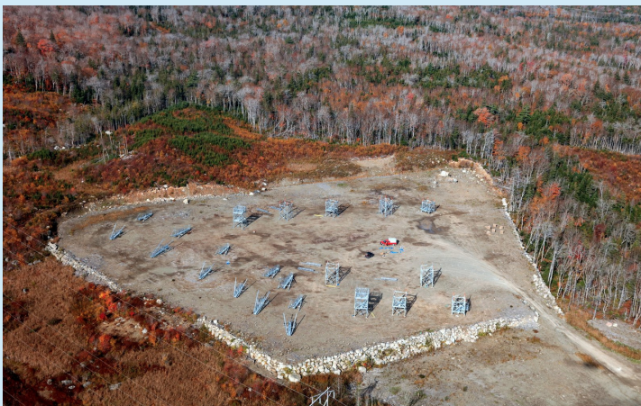
This photo represents a sample assembly yard (Valard Construction)
