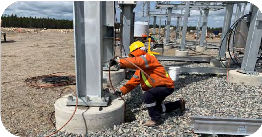
A substation crew member attaches a grounding wire to a structural steel post at the Pipestone Station on NORT Road. All above-ground structures and equipment at a substation need to be grounded for safety and electrical reliability. Underneath the station’s gravel is a network of grounding wire and rods called a “grounding grid” that the copper wire shown in this photo is connected to.
