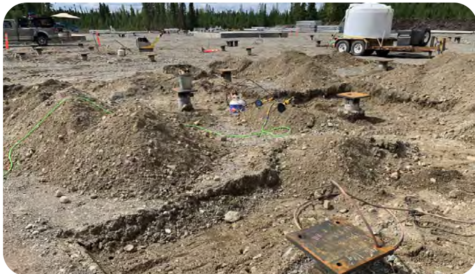
A substation crew member attaches a grounding wire to a structural steel post at the Pipestone Station on NORT Road. All above-ground structures and equipment at a substation need to be grounded for safety and electrical reliability. Underneath the station’s gravel is a network of grounding wire and rods called a “grounding grid” that the copper wire shown in this photo is connected to.
