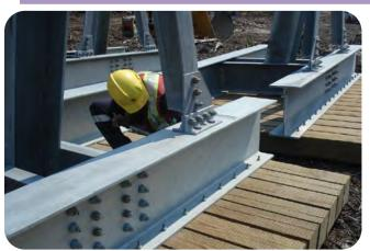
A worker checks the torque of a tower foundation on recently assembled timber mats as part of the quality assurance process. Each bolt needs to be checked before the foundation is buried!
