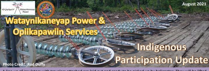
A line-up of insulators with travelers attached are laid out and ready to be picked up by helicopter. They will be lifted to stringing crew members and hung on the "arms" of each structure. The red "fly arms" are designed to be highly visible. The purpose of the "fly arms" is to create a large target for the placement of the pilot rope that is flown by a helicopter. The pilot rope is then used to pull the conductor through the travelers.
