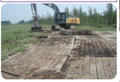
An example of some of the JV work occurring on the Project! An excavator with a grapple lays out temporary matting at a site toward Kingfisher Lake First Nation. The matting protects the land from excessive rutting and allows access to softer areas.
