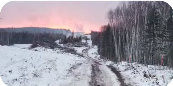
Obish Construction – Segment PQ Line Clearing
