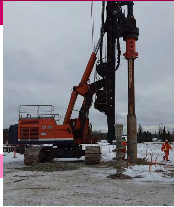
Drilling foundations at the Pickle Lake substation site.
