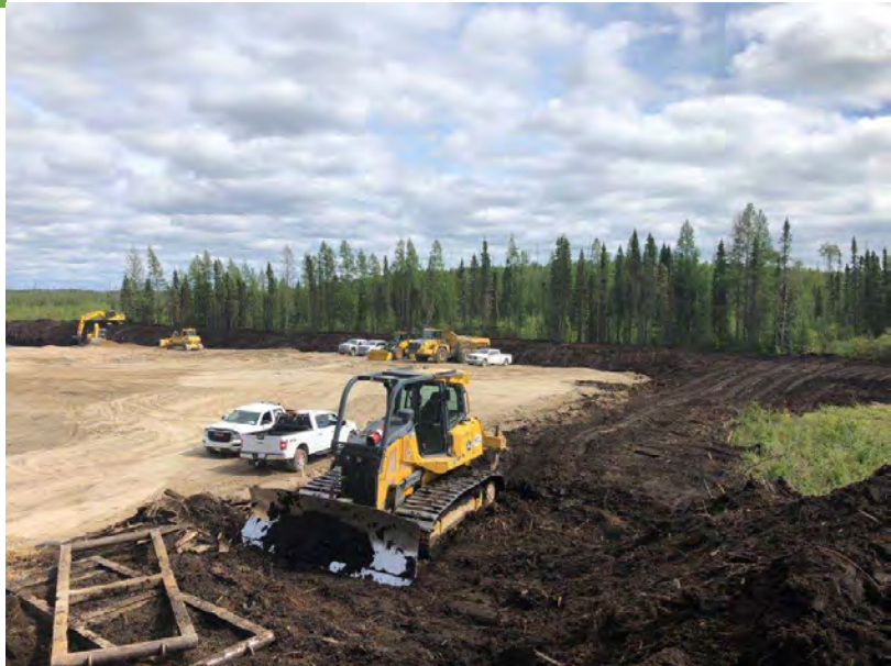
Packing topsoil around the perimeter of the Pickle Lake Substation B.
