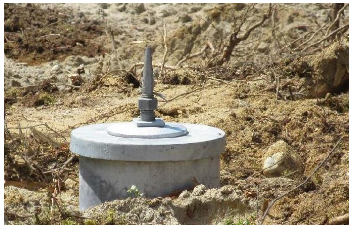
Top of lattice steel tower foundation (pin joint).
